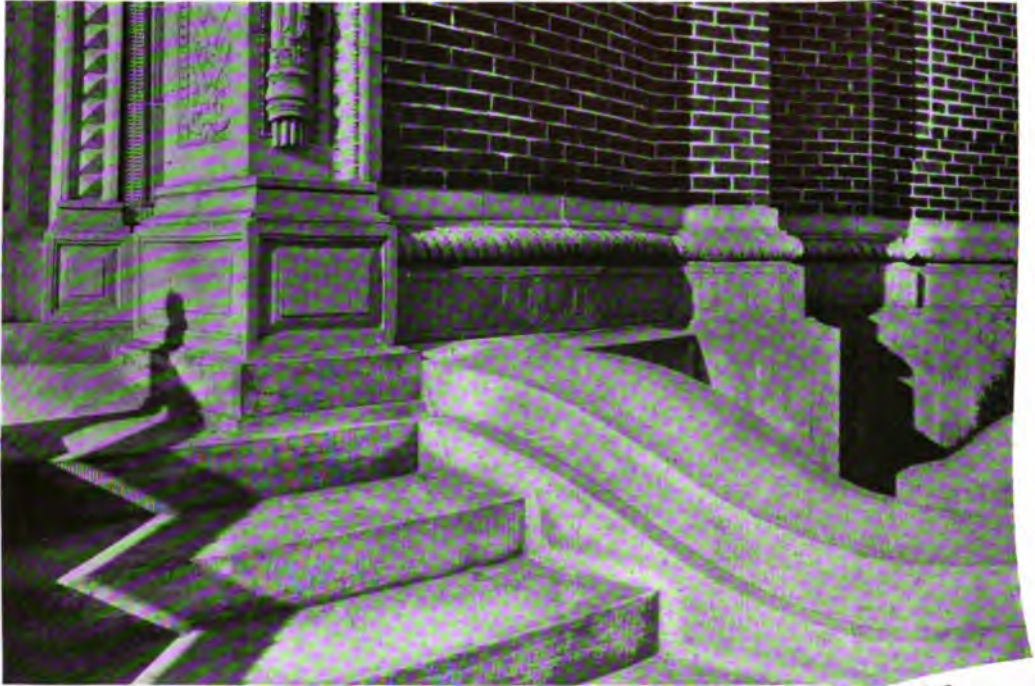
DETAIL AT MAIN ENTRANCE—HADDINGTON BRANCH OF THE FREE LIBRARY OF PHILADELPHIA. Albert Kelsey, Architect.
