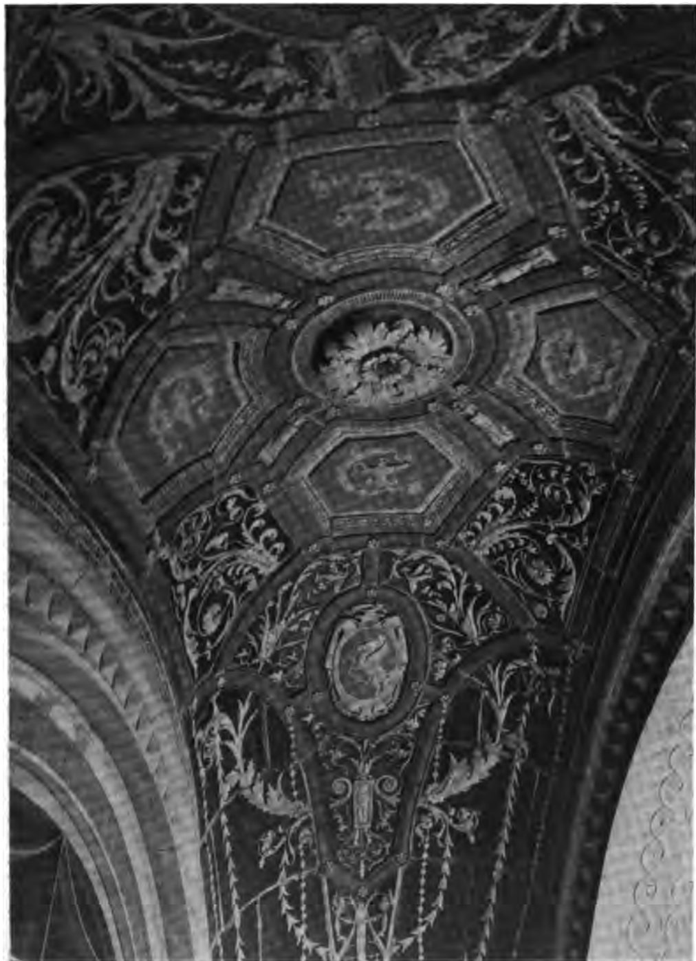
DETAIL OF CEILING IN MAIN ENTRANCE—HADDINGTON BRANCH OF THE FREE LIBRARY OF PHILADELPHIA. ALBERT KELSEY, ARCHITECT.
